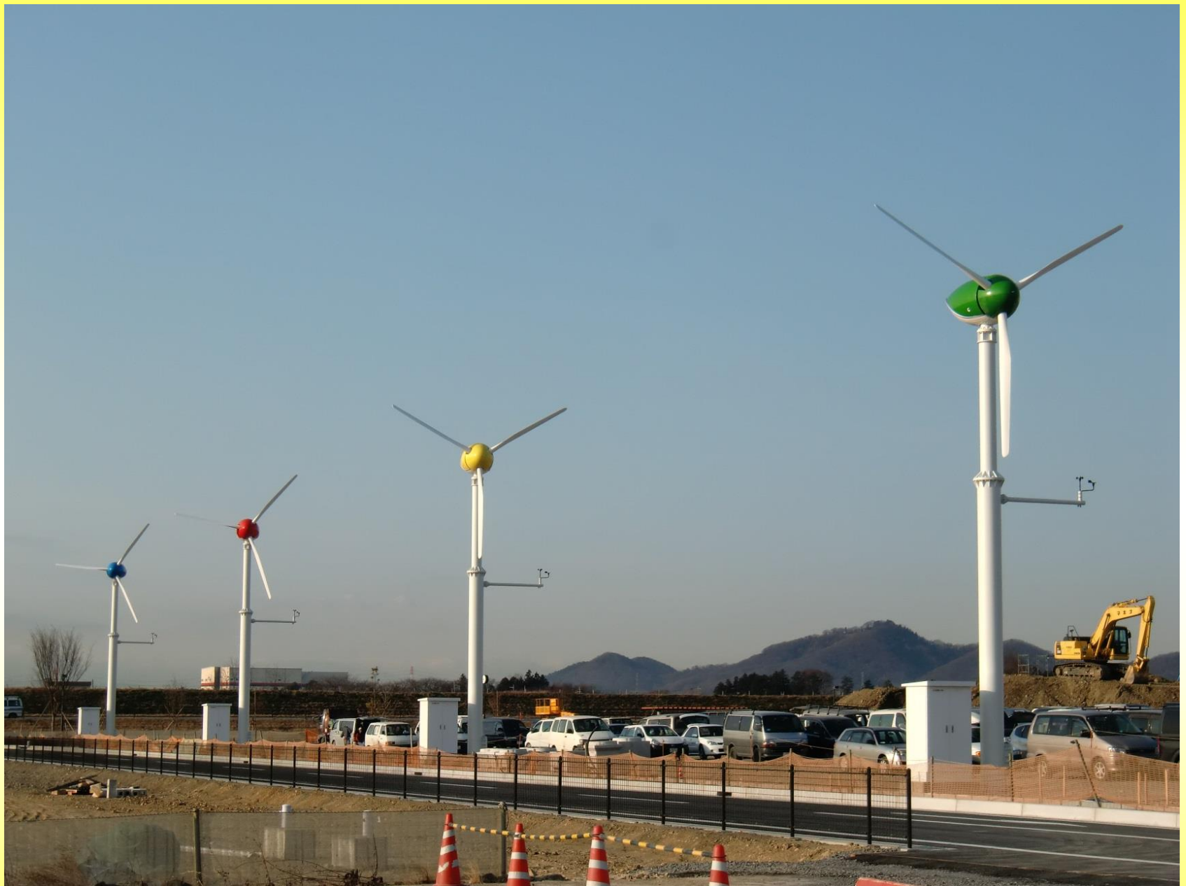
Small Wind Turbine at Ashikaga Red Cross Hospital
