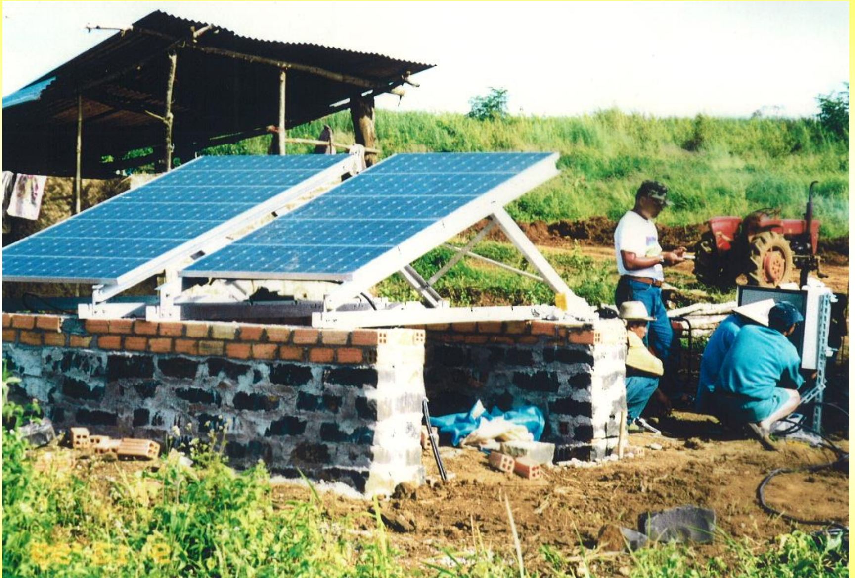
Installed PV Panel
